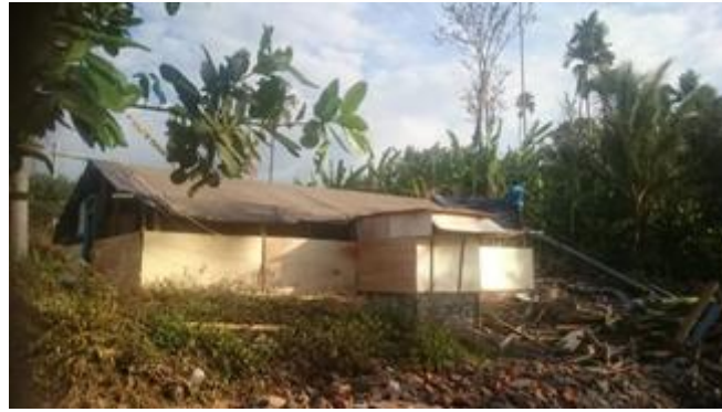
The temporary Mosque moved to semi-permanent building
