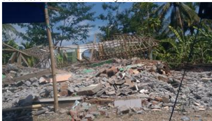
Collapsed Mosque at Tenggorong Hamlet
