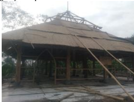
Building the Bamboo Mosque
