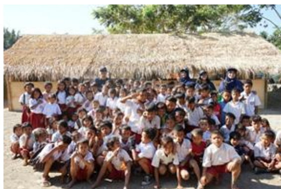
Semi-permanent school building for SDN 04 Gumantar
