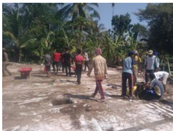
Process of building the Bamboo Mosque
